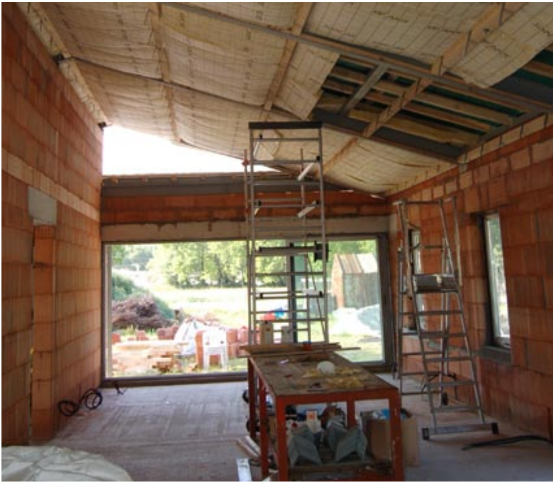
LIVING ROOM INSULATION WORKS PHOTOGRAPHY
