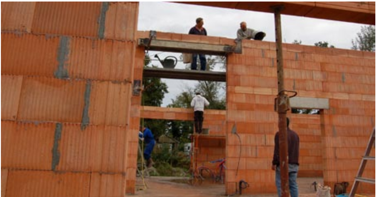
WALLS CONSTRUCTION PHOTOGRAPHY
