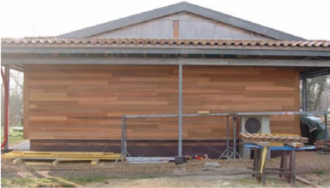
NORTH TIMBER CLADDING WORKS PHOTOGRAPHY
