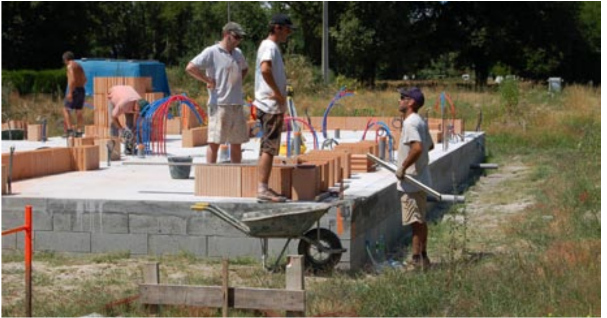
WALLS CONSTRUCTION PHOTOGRAPHY
