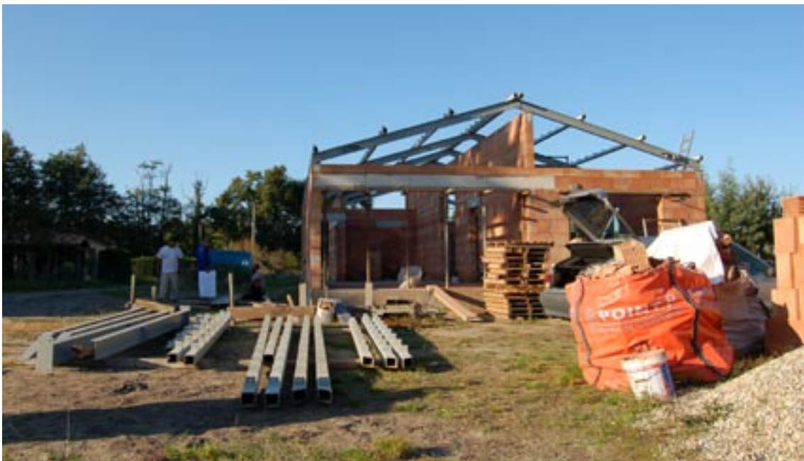
SOUTH STEEL FRAMEWORK PHOTOGRAPHY
