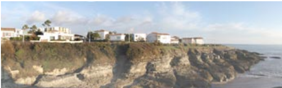
SITE, EXISTING BUILDING PHOTOGRAPHY
