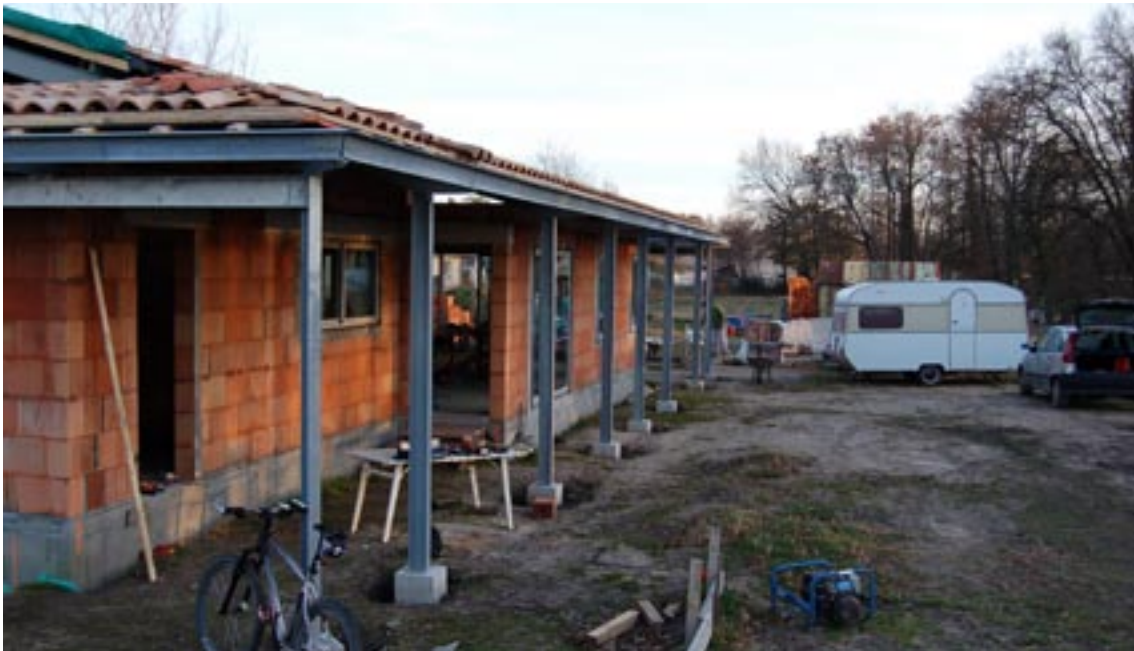
WEST WINDOWS WORKS PHOTOGRAPHY
