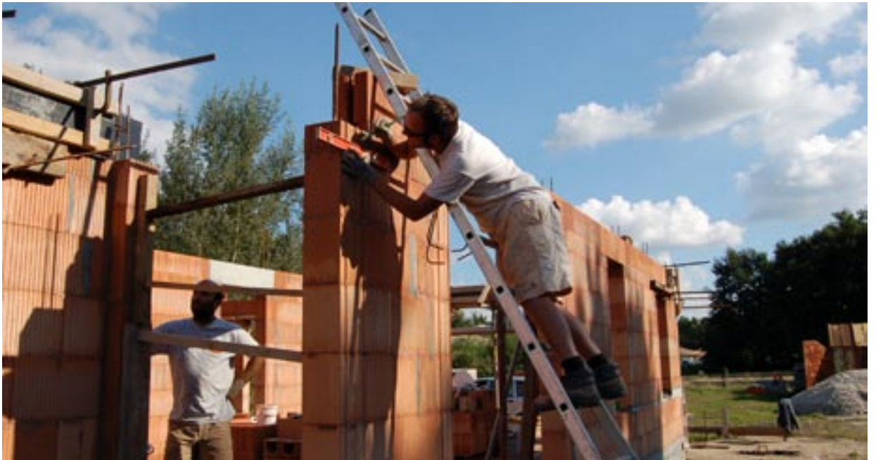
WALLS CONSTRUCTION PHOTOGRAPHY
